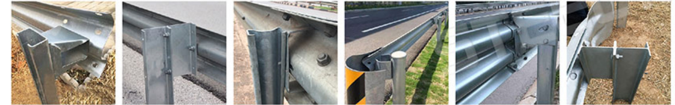
C Post U Post Σ-Sigma Post Round Post Square Post H Post
